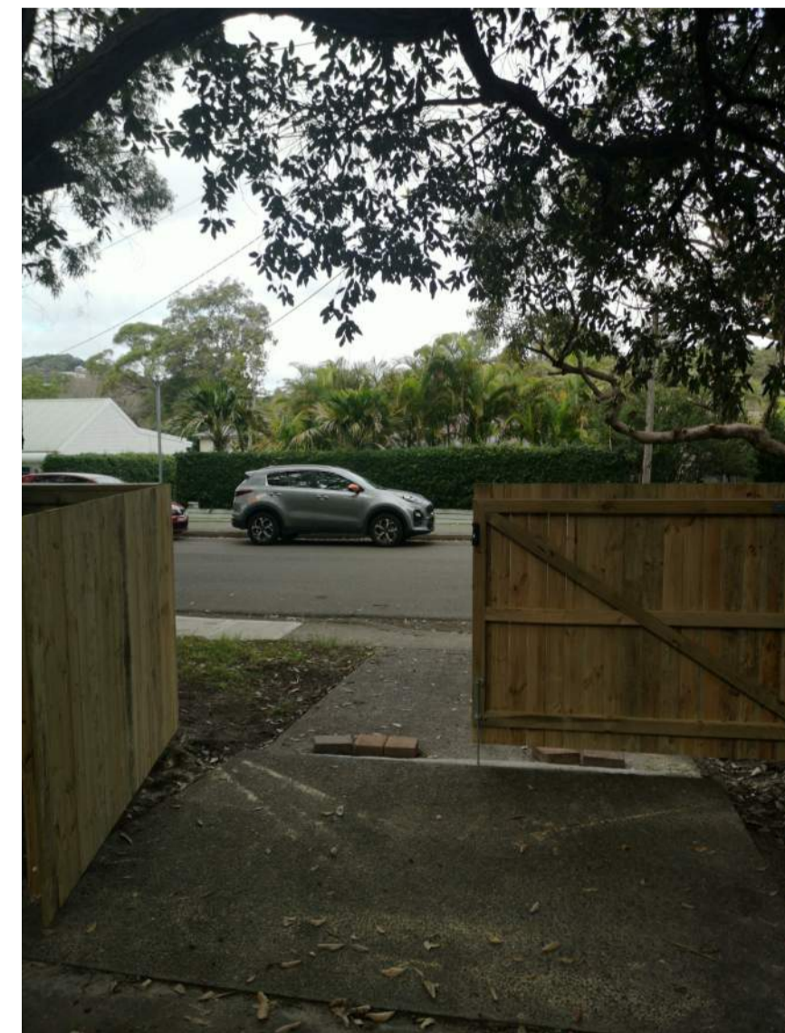
08. EXISTING DRIVEWAY LOOKING AT BARDO ROAD
