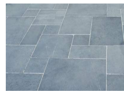
10 ENTRANCE PAVERS BLUESTONE TILES
