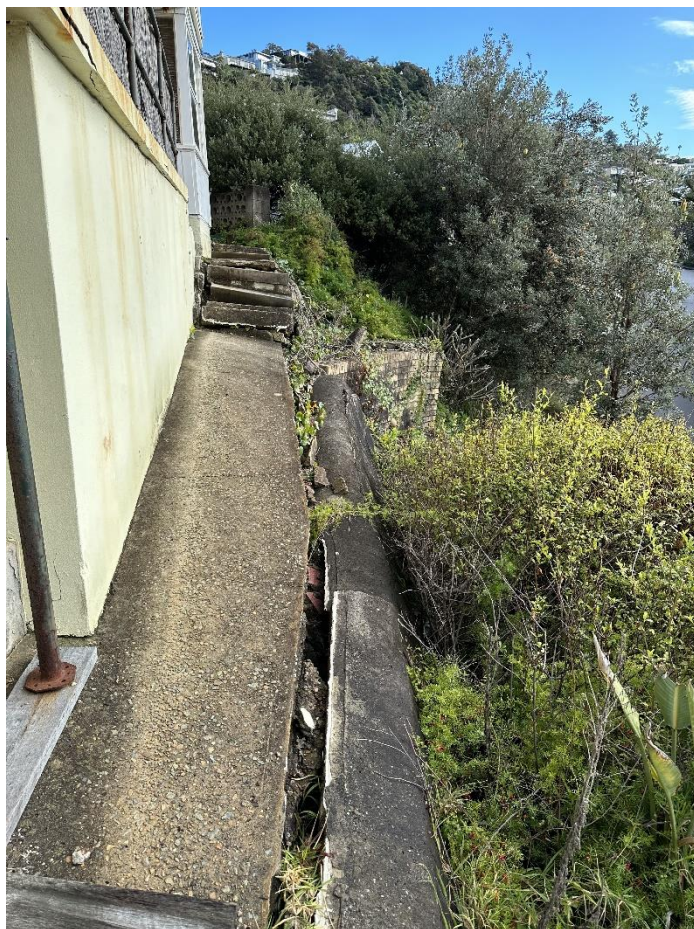
Photo 1 – View of cracking along the external footpath
