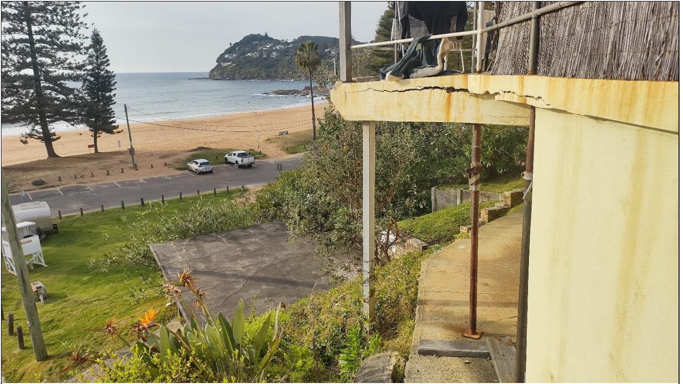
Photo 3 – View of the cracking in the balcony at the eastern side of the site
