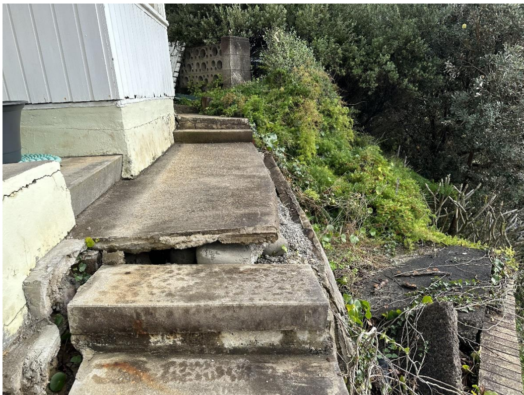
Photo 2 – View of cracking along the external stairs I
