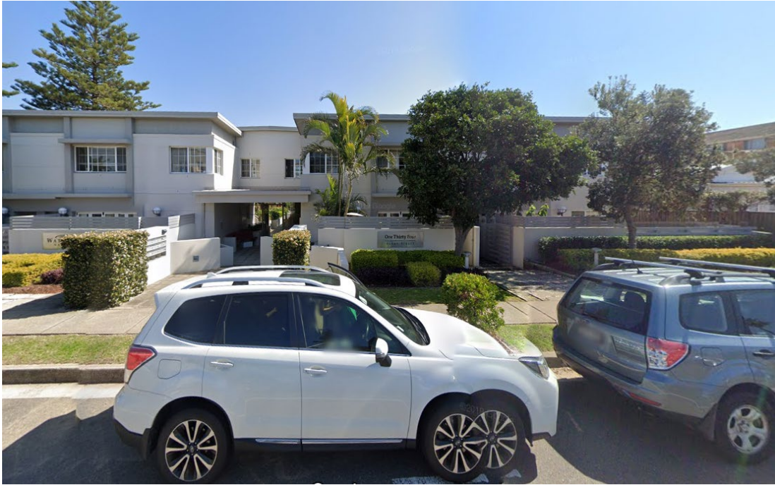
Figure 5 View of adjoining development to the south of the site along Ocean Street Source: Google Maps
