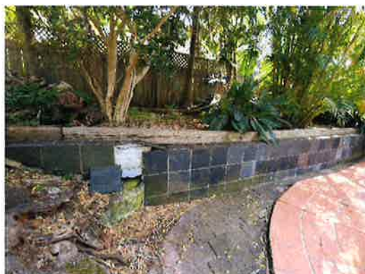
Photograph-12: Concrete tiled retaining wall. View Looking north.
