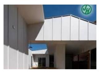
FC WALL CLADDING WITH VERTICAL BATTEN DETAIL (EXISTING RESIDENCE AND GARAGE DOOR)
