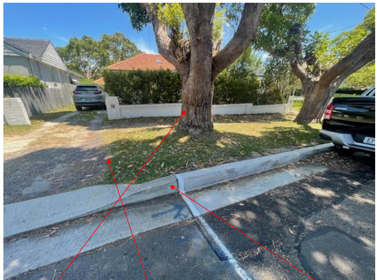
Image A: Tree 1. The existing crossover is compacted therefore should have minimal impact on the tree providing the existing setback is maintained. The kerb and gutter has recently been replaced indicating no additional impacts should be required.
