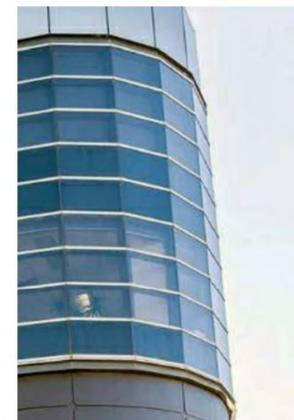
ED-02 CURTAIN WALL MATCH NEIGHBOURING BUILDING WITH A MIXTURE OF DARK TINTED GLASS PANELS (GL-01) AND OPAQUE PANELS (GL-02)
