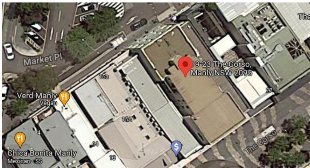
Figure 1: Existing Structure, sourced from Google Maps.
