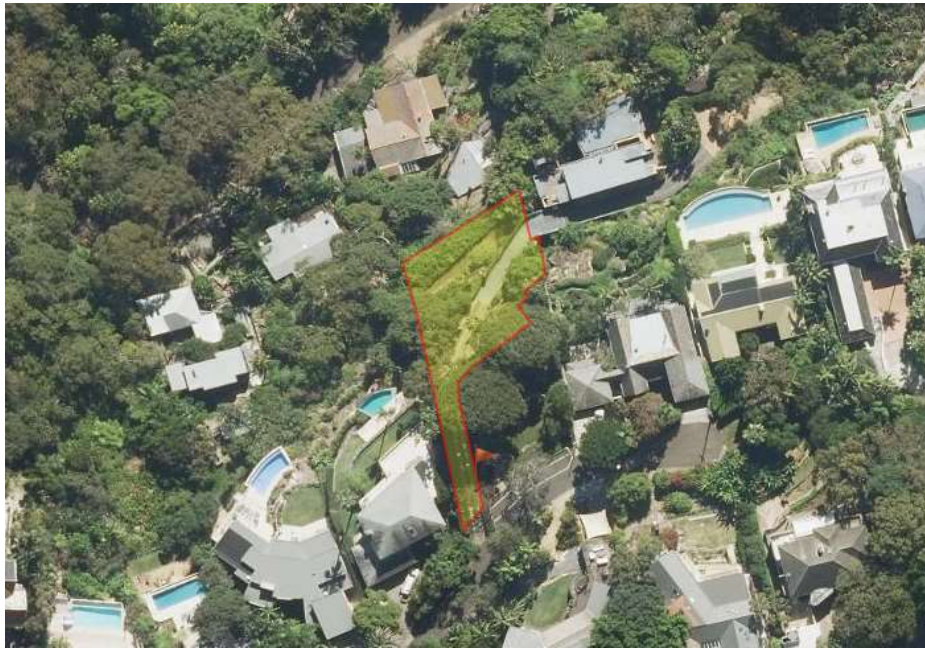
Photograph 1: Aerial photo of site and surrounds
