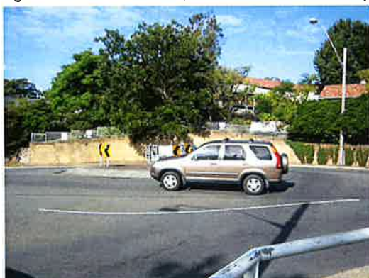
Figure 5.1: McIntosh Road/Fisher Road roundabout (facing west)
