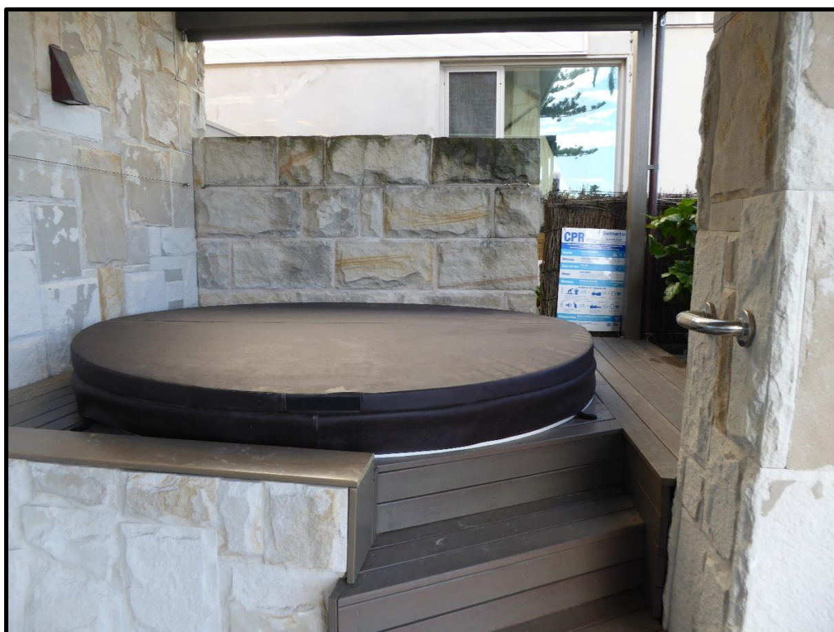
View of spa showing timber surrounds, masonry wall and retractable privacy screens
