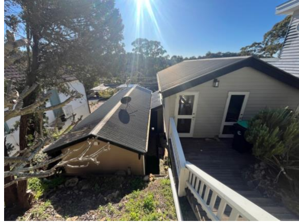
Photo 2: Rear of split two storey dwelling
