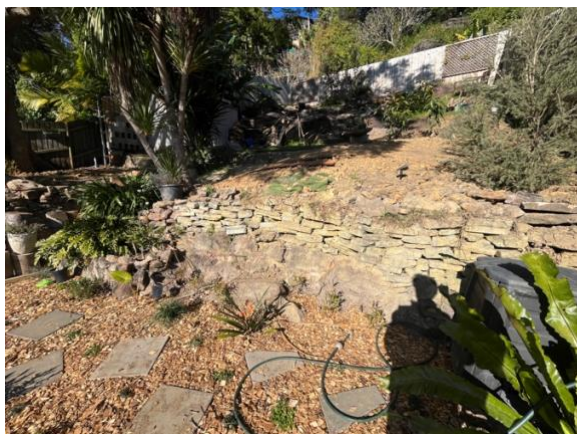
Photo 5: Landscaping wall awaiting completion
