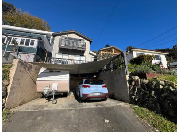
Photo 1: Site frontage, showing existing garage and clad dwelling
