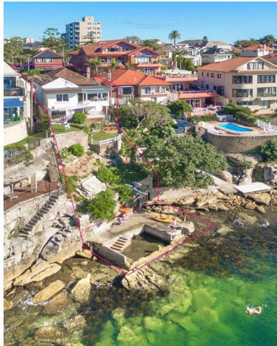
Figure 2: 16 Addison Road Manly – swimming pool located well below the escarpment
