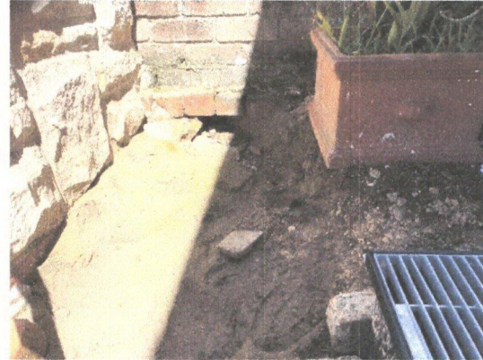
Photo: 2 – Eroded channel below wall
