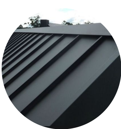
RF - Proposed Roofing Monument - Colorbond To suit 3 degree pitch Gutters, Cappings & Flashings. Refer Hydraulic Plans for sizes & spec
