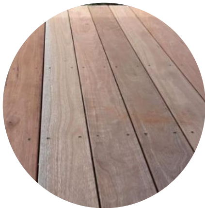
TM - Timber Decking External Balcony Spotted Gum or similar hardwood Sealed, Stainless steel fixings
