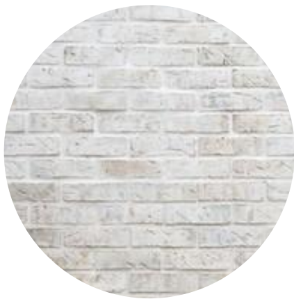
BR - External Cladding Reclaimed Bricks Light bagged render to surface. White wash Paint finish -
