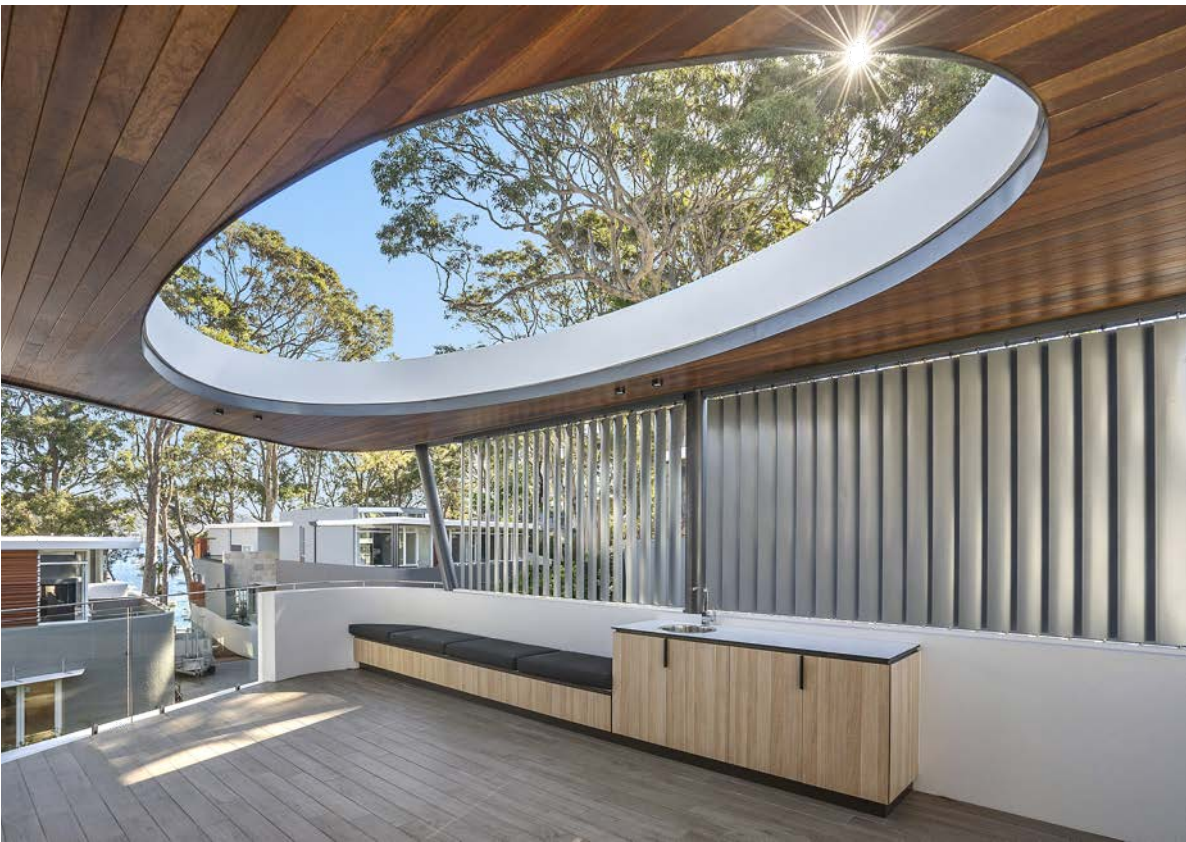
1 PROPOSED PRIVACY SCREENS ADJUSTABLE VERTICAL BLADES
