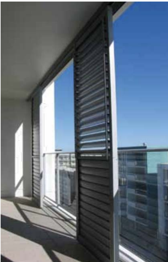
2 PROPOSED PRIVACY SHUTTERS STACKING PANELS WITH ADJUSTABLE HORIZONTAL BLADES
