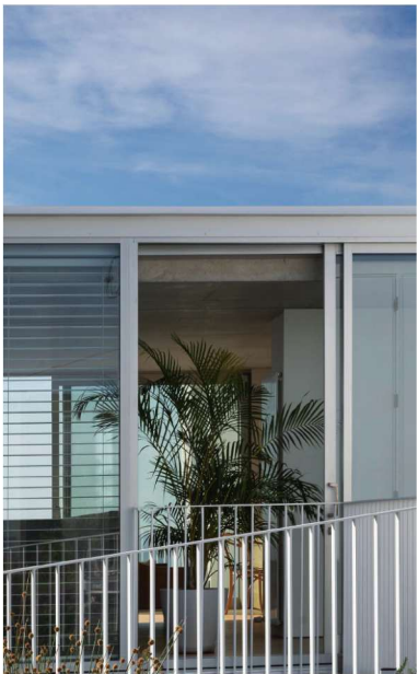
AG.02 - ALUM. GLAZING Powdercoated aluminium with clear glazing
