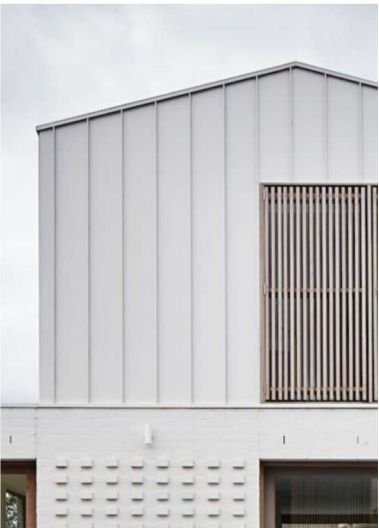
CL.01 - VERTICAL CLADDING White painted cladding
