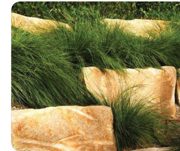
Sandstone retaining walls
