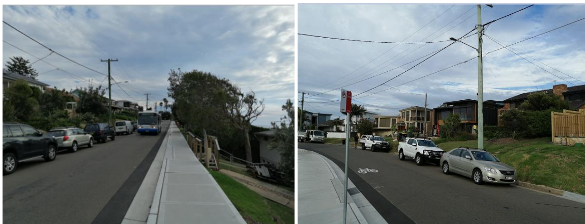
Figure 1: Regular Bus Route on Narrabeen Park Parade and No standing or stopping on the Eastern kerb.
