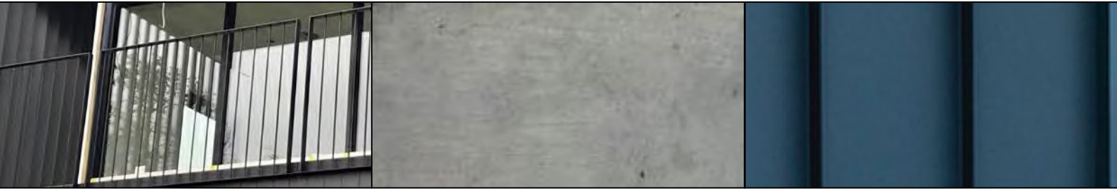
BA. BALUSTRADE VERTICAL BARS POWDERCOATED MATT BLACK DR. DRIVEWAY CONCRETE TROWLED RO. ROOF - METAL STANDING SEAM MATT BLACK OR SIMILAR
