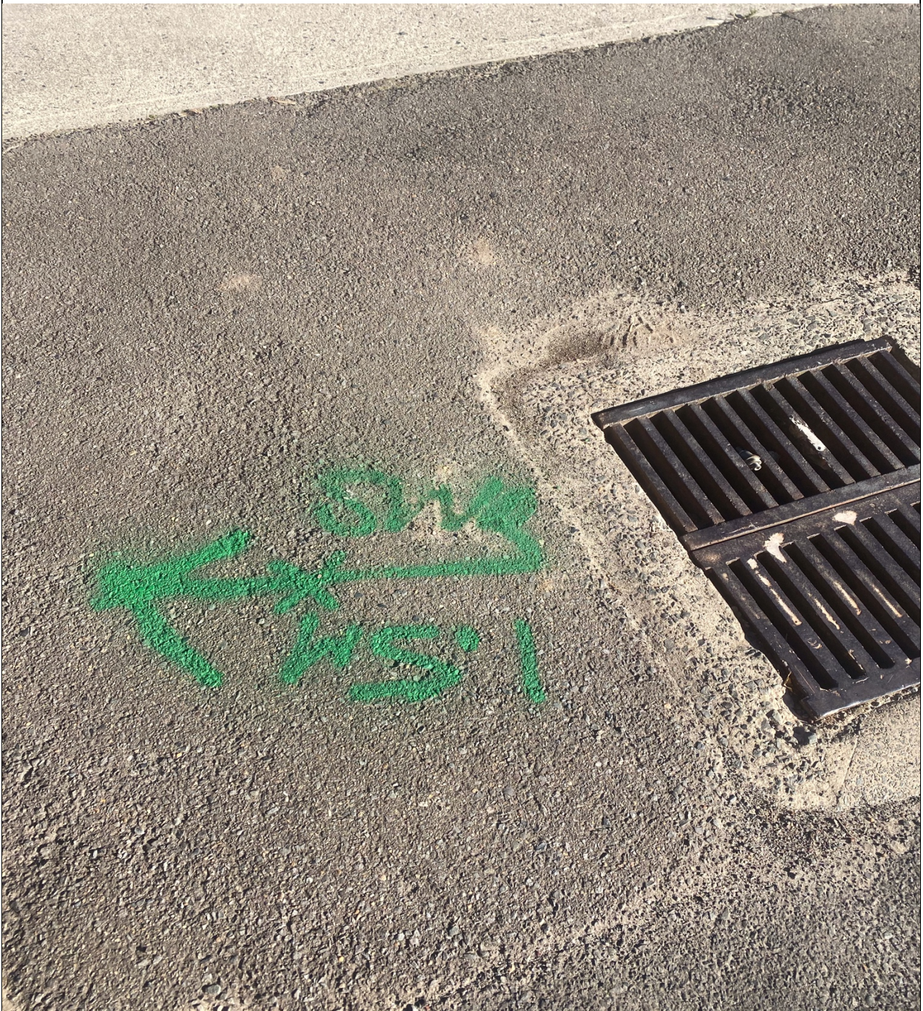
Pit at corner of large shed:
