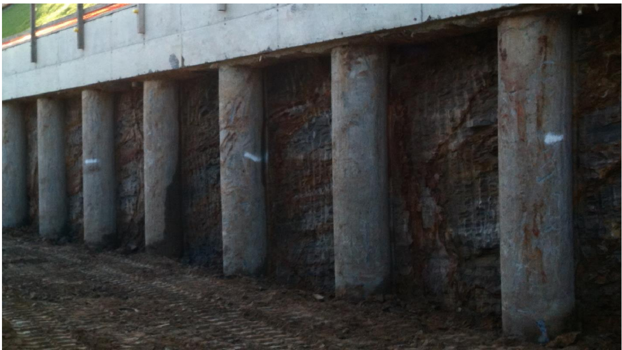
Figure 3, geological conditions behind soldier pile retaining wall on eastern boundary prior to placement of shotcrete infill.
