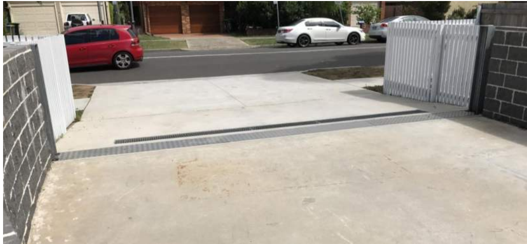
Figure 2: Flood barrier at 1 Mactier Street, Narrabeen, NSW in down position.
