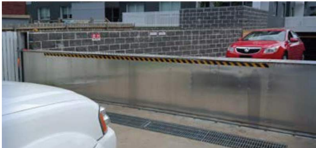
Figure 3: Flood barrier at 1 Mactier Street, Narrabeen, NSW in up position.
