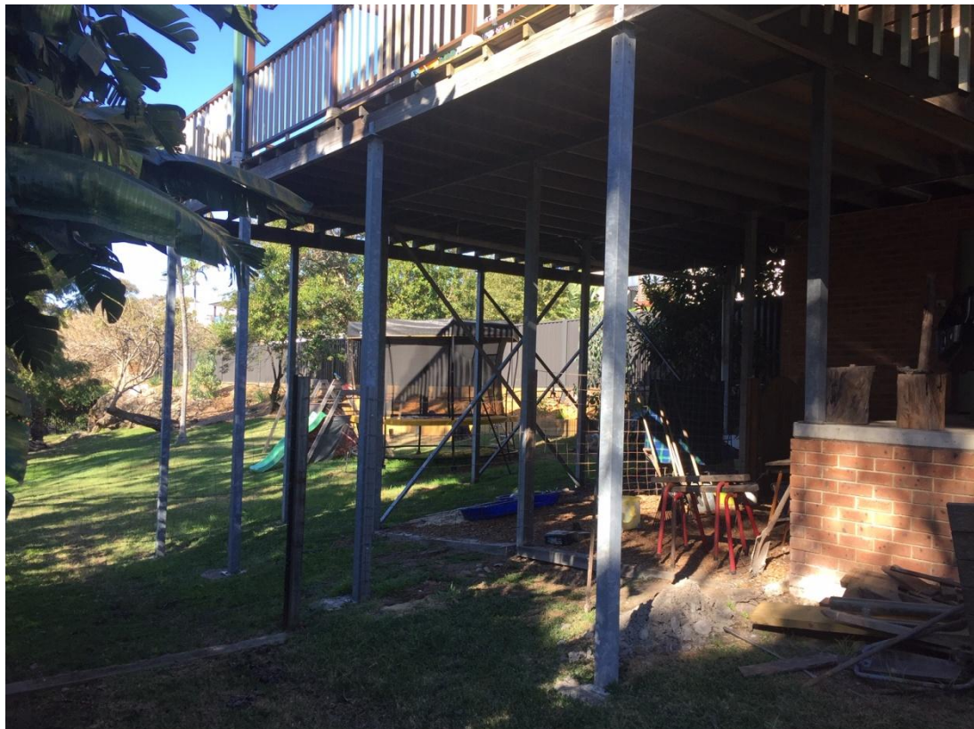
PHOTO No 10 – Underfloor steel columns and cross-bracing
