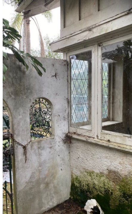
Figure A.5 Southeast corner with leadlight and replacement windows. Rising damp typical of all walls. (Source: Skerrett, 2020)
