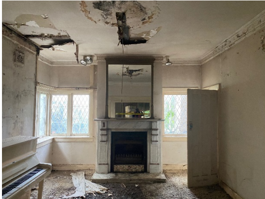
Figure A.6 Living room with reproduction chimney piece and fallen rose (not original). Unsafe floor and ceiling. (Source: Skerrett, 2020)
