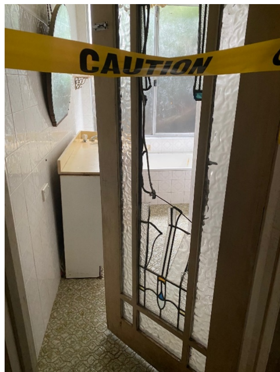
Figure A.9 Modern refurbished bathroom inserted as part of alterations and additions at north end of west elevation. Damage to original door is typical of vandalism throughout. (Source: Skerrett, 2020)
