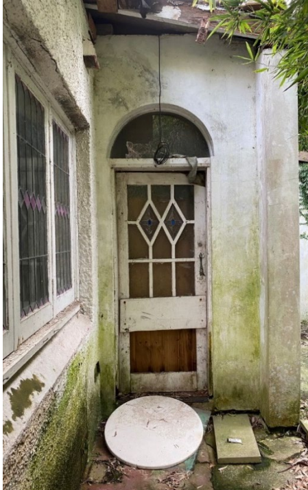
Figure A.4 Northwest corner with damaged and reused door to altered kitchen area. Rising damp throughout. (Source: Skerrett, 2020)
