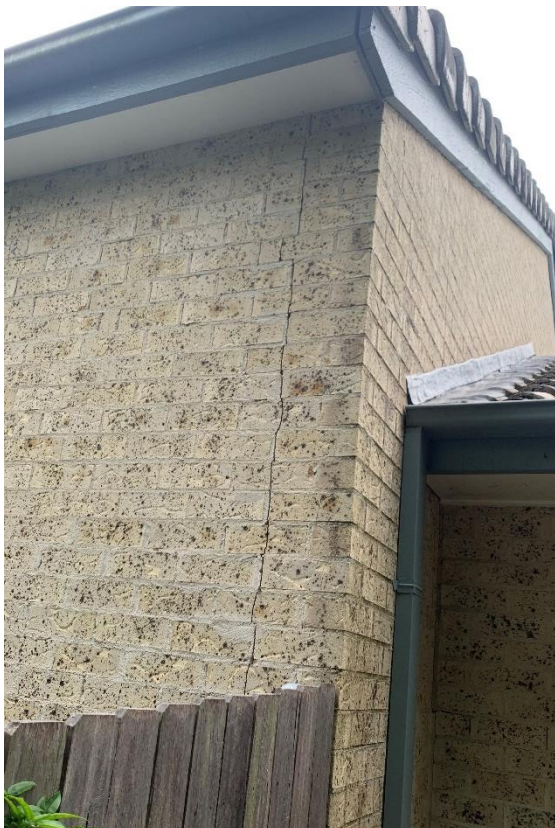
Photograph 3: Vertical crack within rear external wall
