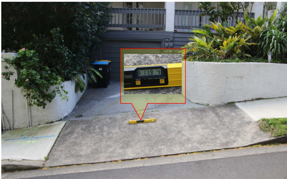
Photo 2.2: Gradient of the current driveway (Photo: traffic Engineering Centre Pty Ltd)
