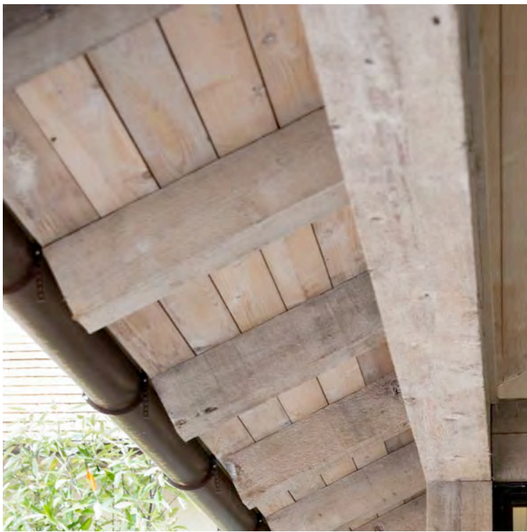
06 WASHED TIMBER EAVES AND SOFFIT
