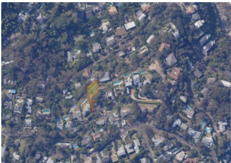
Figure 1.1 Location of the site. Source: Six Maps, 2020.
