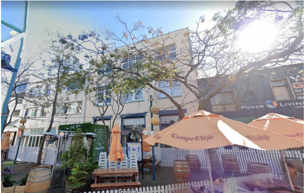
Figure 4: Subject property as seen from Market Place
