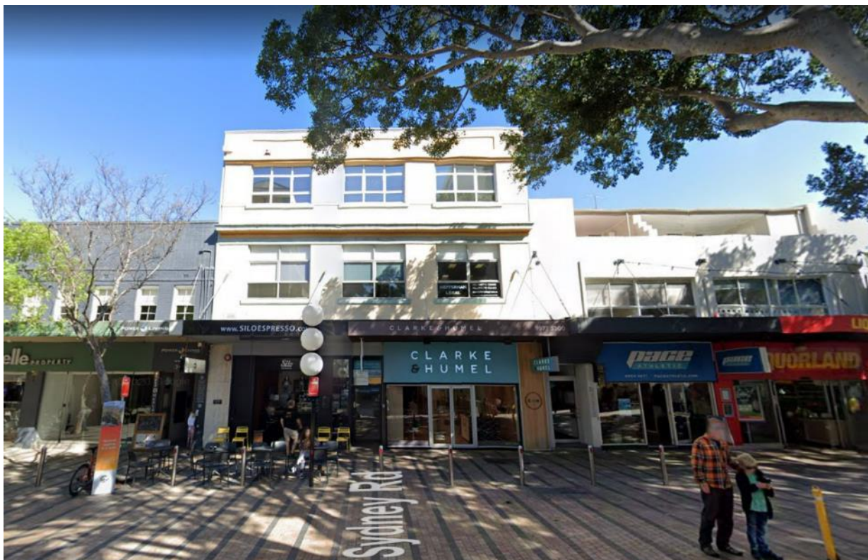
Figure 3: Subject property as viewed from Sydney Road
