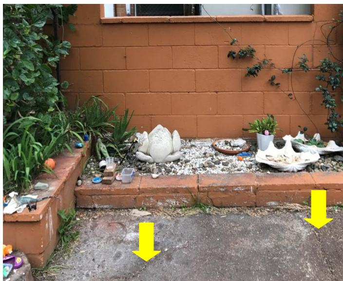
Photograph 4: Cracking in raised courtyard, looking west.
