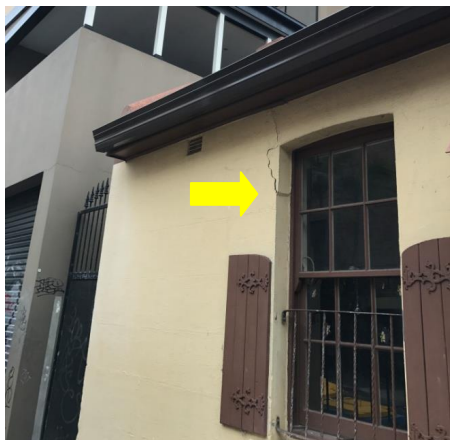
Photograph 3: Observed cracking within the front wall of the dwelling, looking west.
