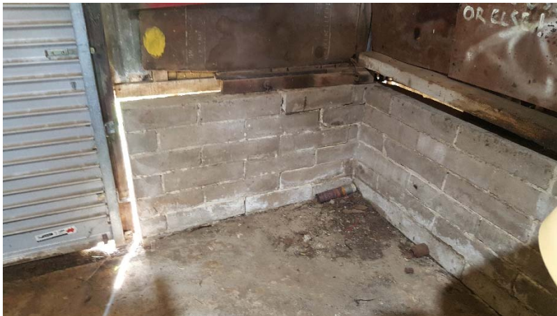
Frame 1 – Brick retaining wall found to be stable / in good condition and structurally adequate.
