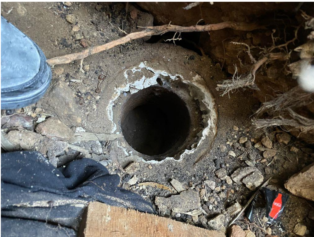
Above: Recent photo on site showing existing sewer pipe connection at ground – a camera in the pipe showed it in good condition, clear of blockages and available for connection.
