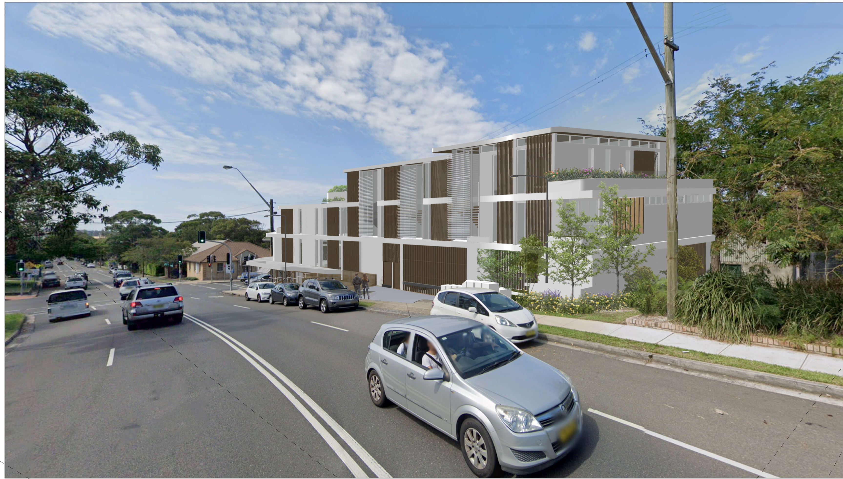
GREEN ELEMENTS SUCH AS BALCONY PLANTERS & CLIMBERS SOFTEN THE FACADES & PROVIDE VISUAL RELIEF
