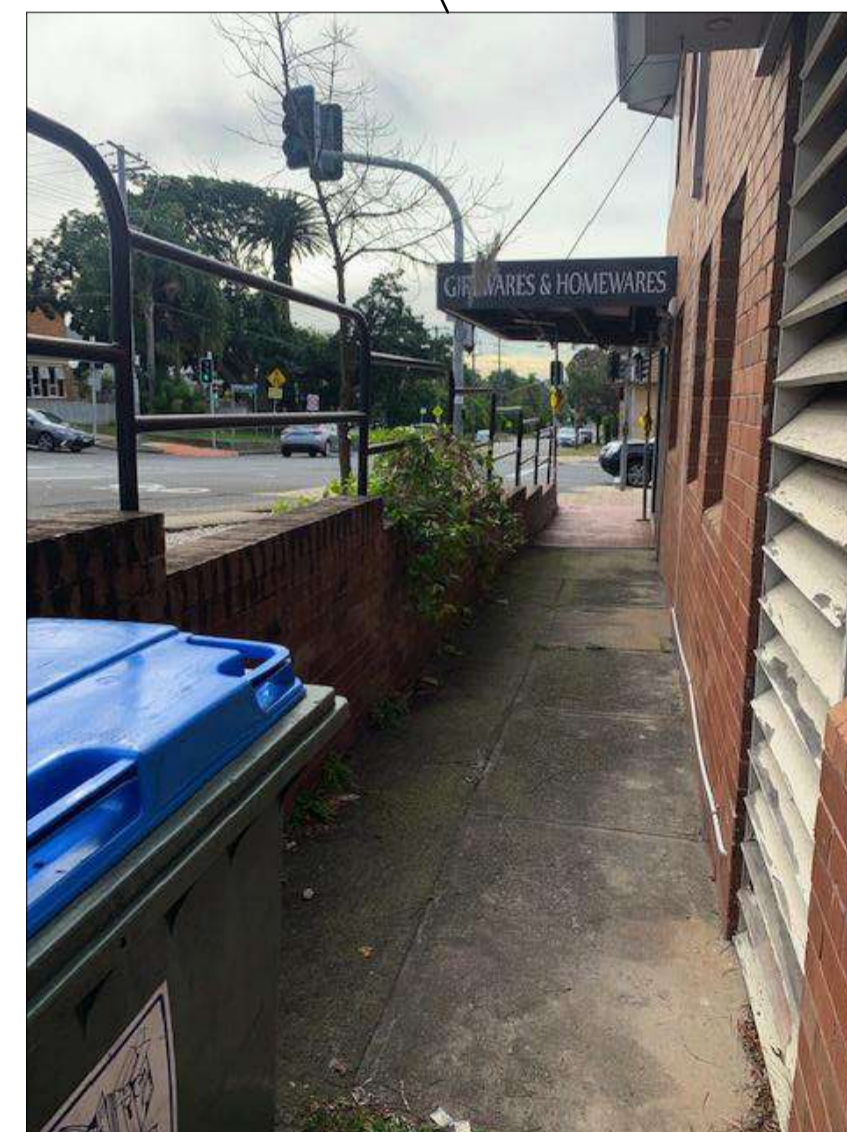
EXISTING RETAINING WALL ALONG OLIVER STREET TO ACCOMMODATE THE SLOPE OF THE ROAD. SIMILAR APPROACH USED WITH THE PROPOSED SCHEME FOR THE OUTDOOR SEATING AREA
