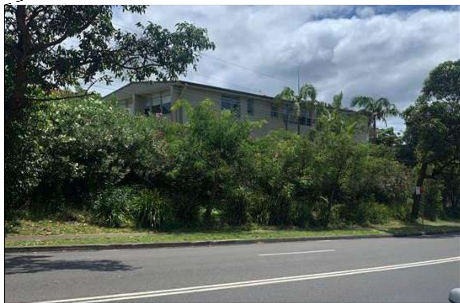
RESIDENTIAL BUILDING ACROSS OLIVER ST TO THE WEST
