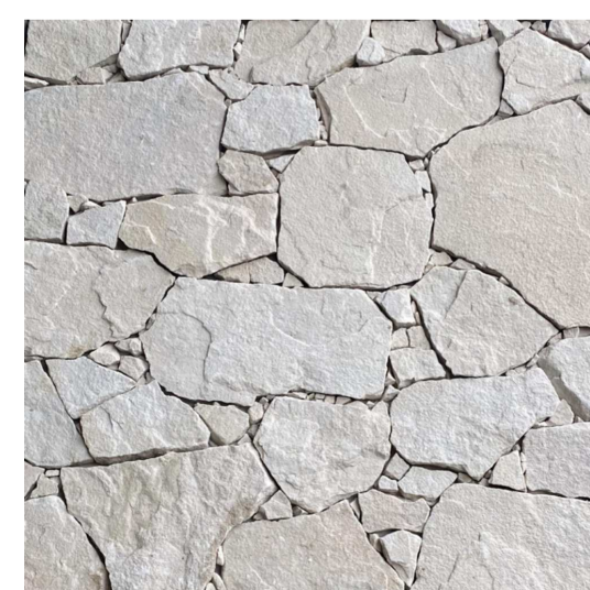
4 Example of stone cladding
