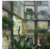
2 GRATING PANELS AND STEEL WIRES WITH SCREEN PLANTING
