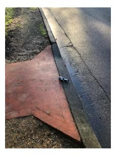
2. The kerb ramp provided on the corner of North Avalon Road and Catalina Crescent (south side of North Avalon Road at the pedestrian crossing) has a gradient that is steeper than 1:8. This is not compliant with the maximum gradient of 1:8 allowed under clause 26 (3)(iii). See photo below. The sections steeper than 1:8 is the orange section in the photo below as well as the grey section. The orange section gradient was approximately 1:5.8 and the grey section was approximately 1:6.5.
