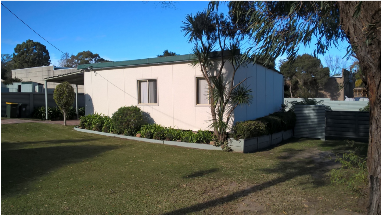
Photographic Plate 19: Rural residential property that is located immediately beyond the eastern boundary of the subject site appeared to be walled with bonded asbestos sheeting, south-eastern perspective
