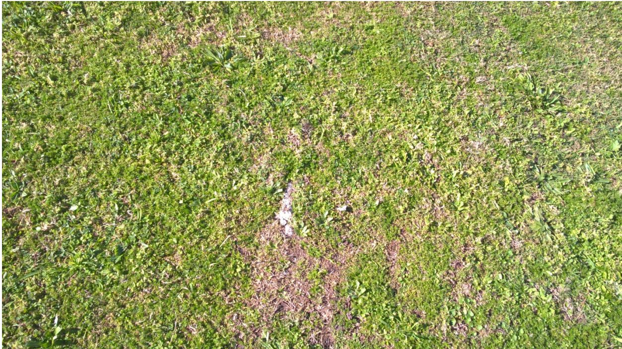
Photographic Plate 15: Concrete fragment within surface soils in south eastern corner of subject site
