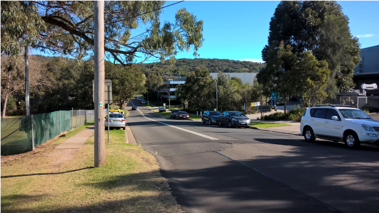
Photographic Plate 3: Light commercial development to the west of the subject site, western perspective from Jubilee Avenue footpath
