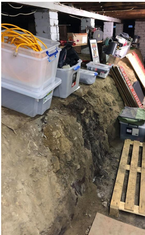
Photograph 9: Stepped soil profile in basement sub floor level, facing south east
