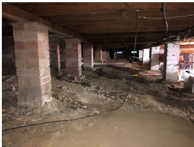
Photograph 10: Exposed footings in basement sub floor level, facing south east
