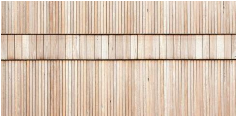
Timber feature battening and/or cladding proposed to be natural blackbutt timber (or timber look) finish (TBC). Timber details including proposed timber screens and gate to be natural blackbutt timber (or timber look) finish (TBC).
