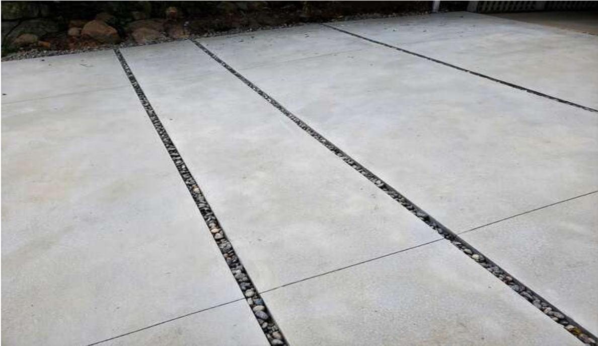
Driveway - Sandblast concrete with gap between slabs
