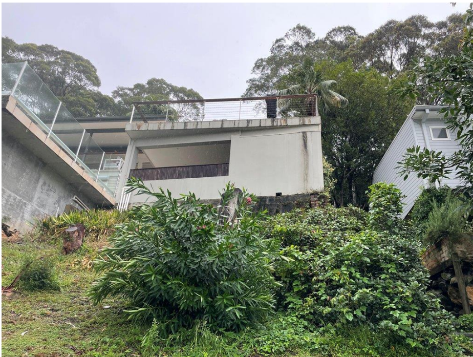
Figure 11 – the existing development as viewed from the rear of the site
