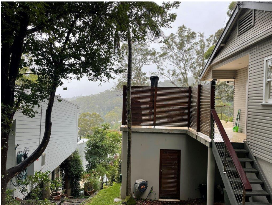
Figure 9 – existing dwelling’s elevated balcony and western setback (Interface)
