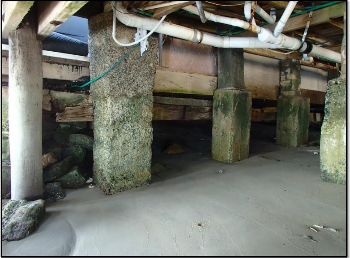
Existing Supporting Piles for Upper Level Deck (Cardno Report)
