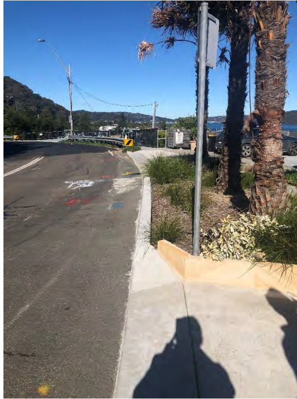
Sandstone seating of reconstructed bus bay
