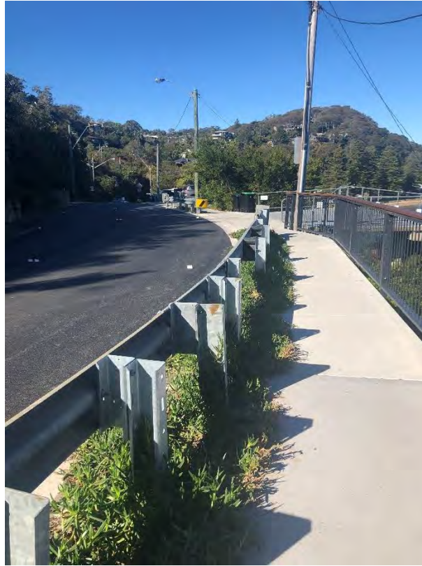
Shortened Barrier to Provide Parking Access to No.1167 Barrenjoey Road
