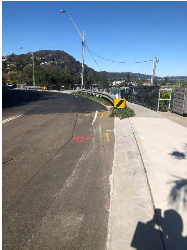
Shortened Barrier to Provide Parking Access to No.1167 Barrenjoey Road
