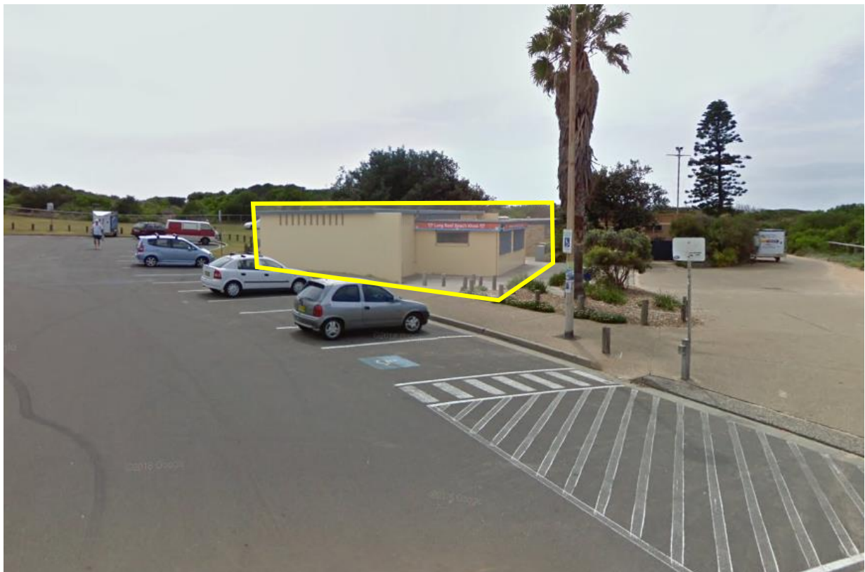
Figure 2 – Development Site viewed from car park, facing east
