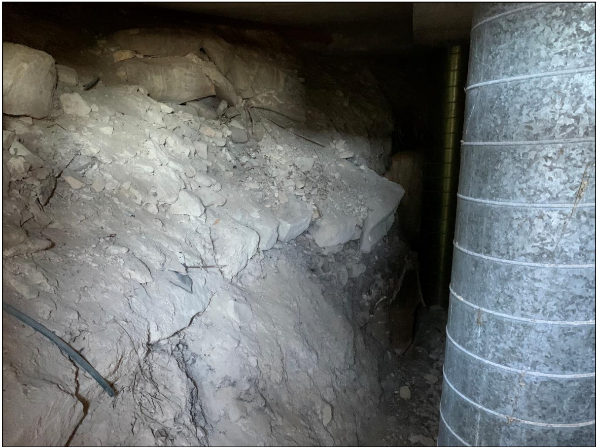
Figure 2 Loose Cobbles on Sandstone Bedrock
