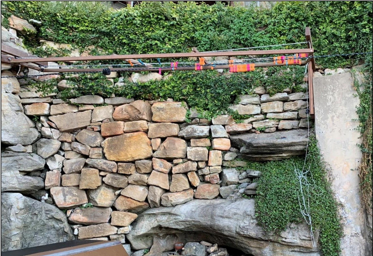
Figure 3 Dry Stone Wall
