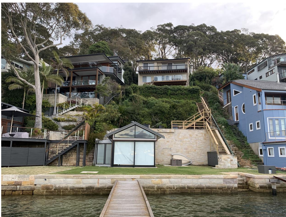
Figure 5 Existing Foreshore fronting 24 Cabarita Rd, Avalon Beach
