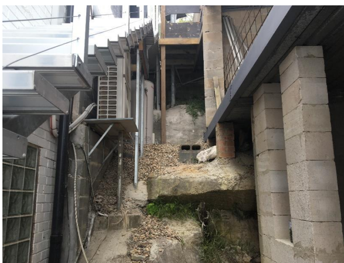
Photograph-6: Level four supported in brick columns directly on to rock, view looking east.
