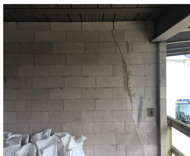
Photograph-9: Vertical crack. View looking
