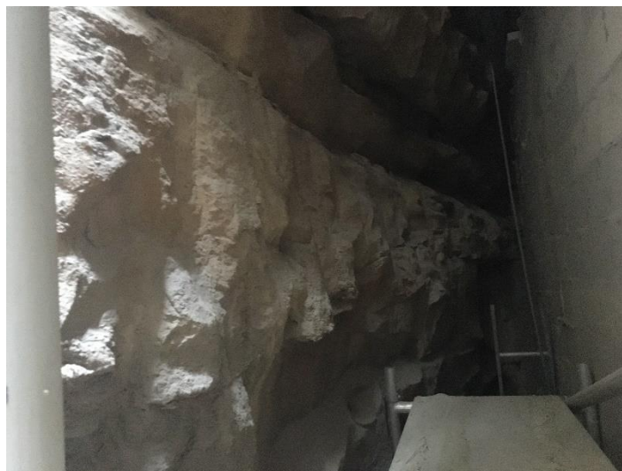
Photograph-15: Steeply defect joints from behind the wall. View looking east.
