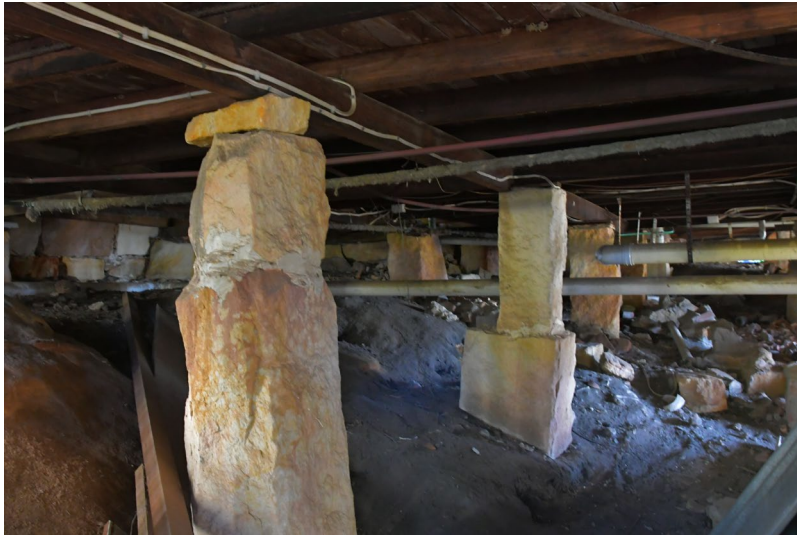
Fig 10 View of house sandstone foundations and services showing adhoc unstable construction.
