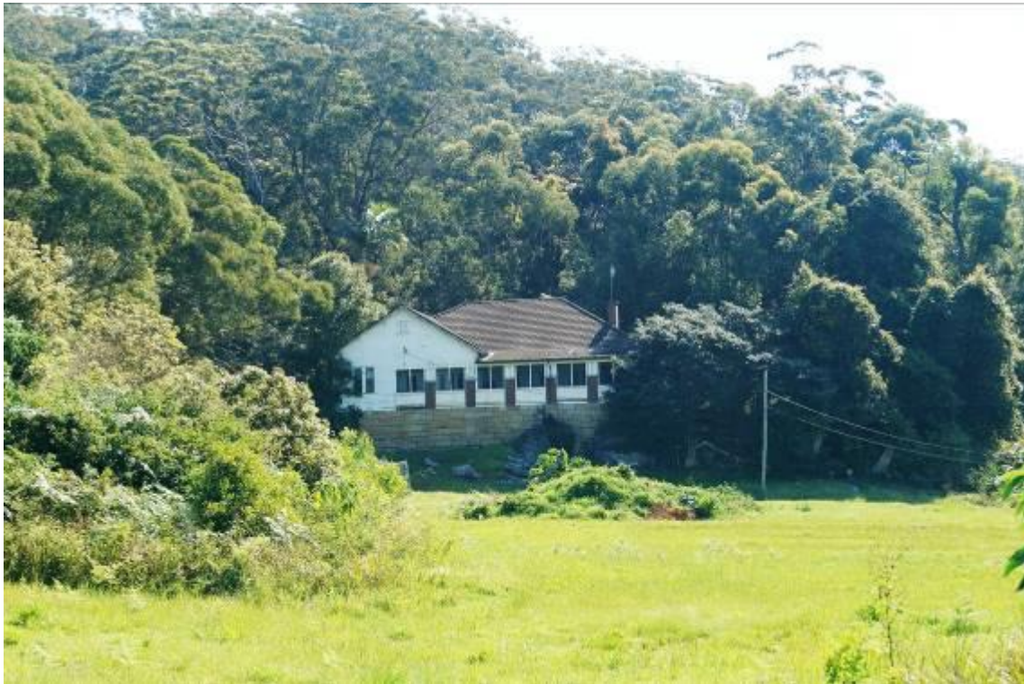
Figure 7 - View looking west from centre of site towards existing dwelling house
